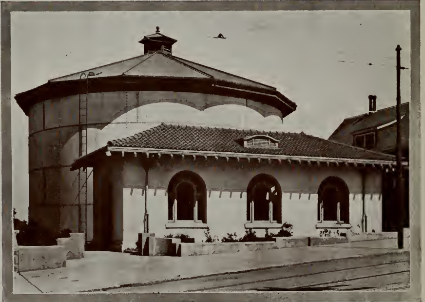
ASHBURY HEIGHTS PUMPING STATION
